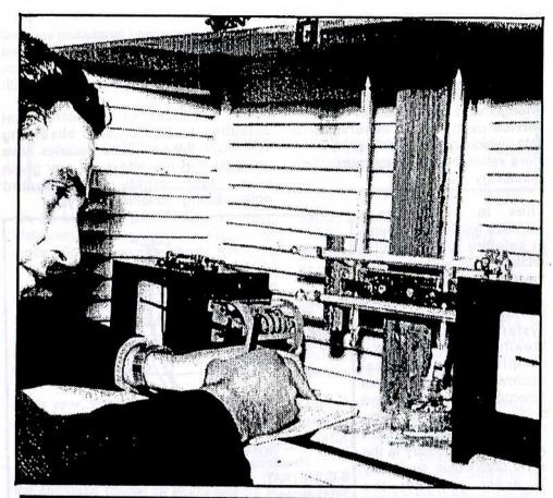
An observer taking temperature and humidity readings at a Stevenson screen. Instruments shown are: wet and dry bulb thermometers(horizontal), bimetallic coil thermogram (at left) and hair hygrogram (relative humidity recorder).
